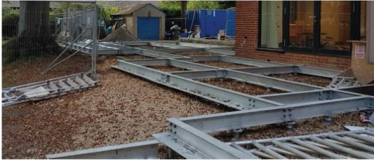
Images indicate Root Bridge structural system, which seating will be installed onto
